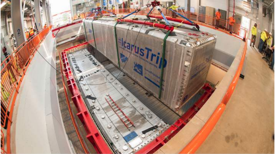
Figure 5.3: ICARUS insulated cold vessels assembly into the warm vessel at Fermilab. Figure provided by the ICARUS collaboration.
