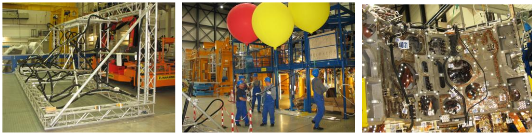
Fig.10 Trial installation of the bus bars on module 4
