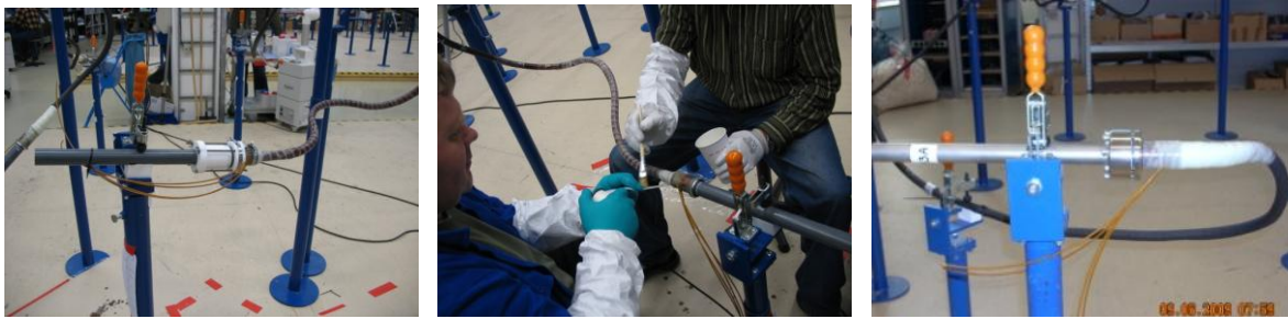
Fig.12 Electrical insulation of bus bar ends at various steps
