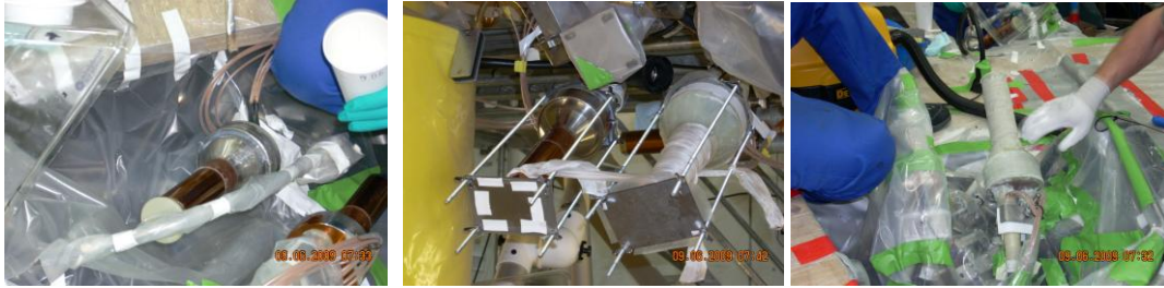
Fig 17. Various phases of joint insulation (mainly wet lamination of glass fibre tapes)
