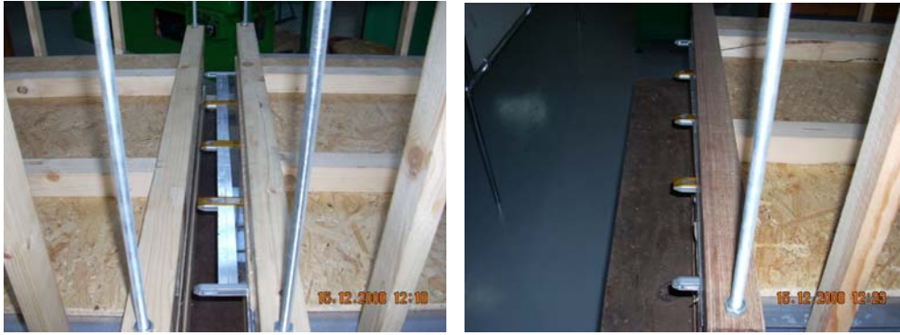
Fig. 18 Tapered ends of extended Al profiles facilitate transition of the modules from one tower to another (left); dummy module in the innermost tower (right)
