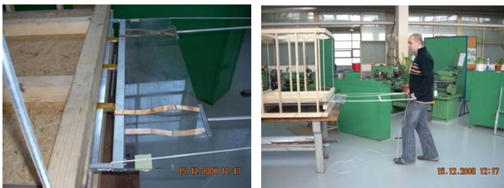
Fig.17 Each segment of the jig enables a transition of the module through one tower
