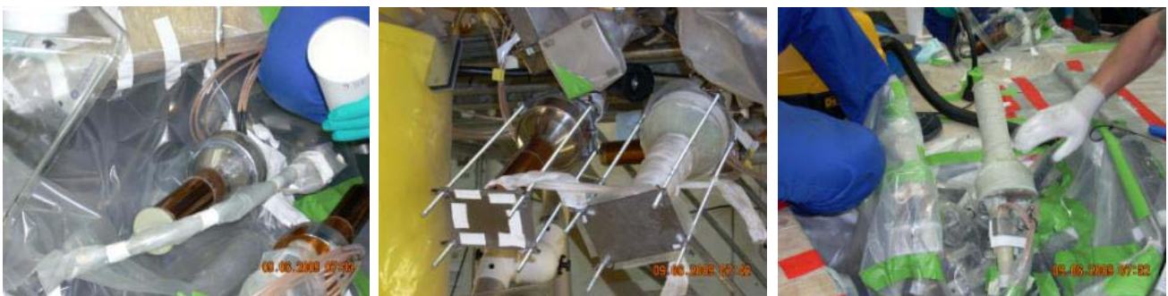
Fig.7 Electrical insulation of joints
