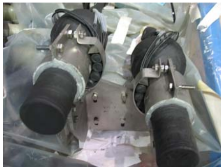
Fig.9 Two joints with QD boxes already painted and fixed
