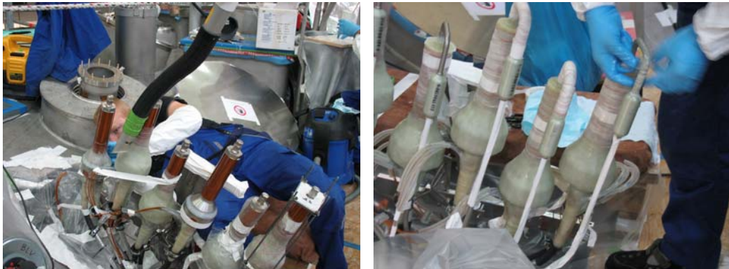
Fig.12 First step of insulation process (left); second step (right).
