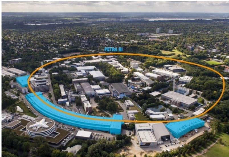
Figure 39 View on the DESY facility with PETRA III synchrotron [22]
