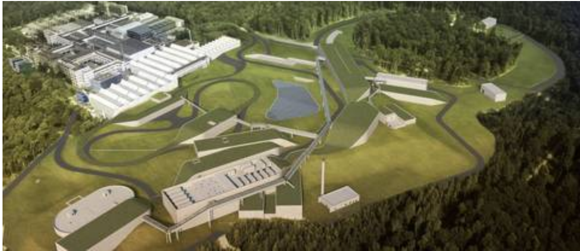
Figure 34. The FAIR facility currently under construction.
